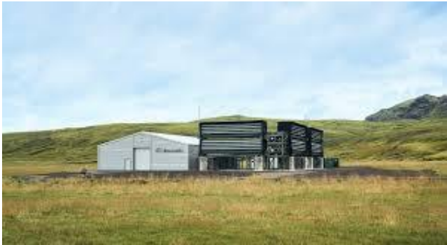
Orca, biggest CO2 Direct Air Capture plant in the world starts operations in Iceland in 2021
