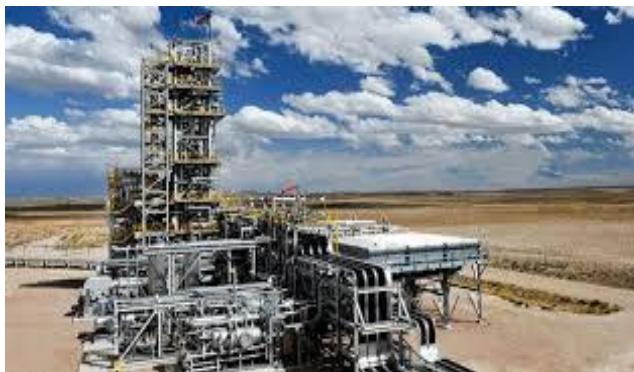
Shute Creek – world’s largest carbon capture facility sells CO2 for oil production, but vents unsold
